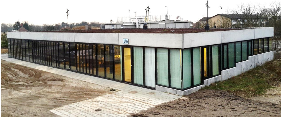
Figure 6-2 WWTP building at Herlev Hospital. The two biological reactors are placed behind the building.
