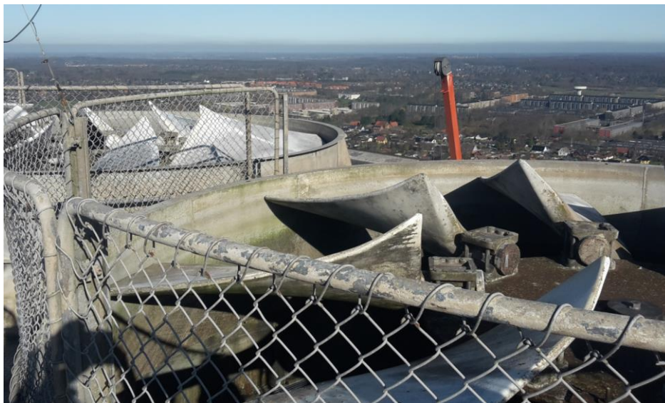
Figure 12-4 Cooling towers at the rooftop of Herlev Hospital
